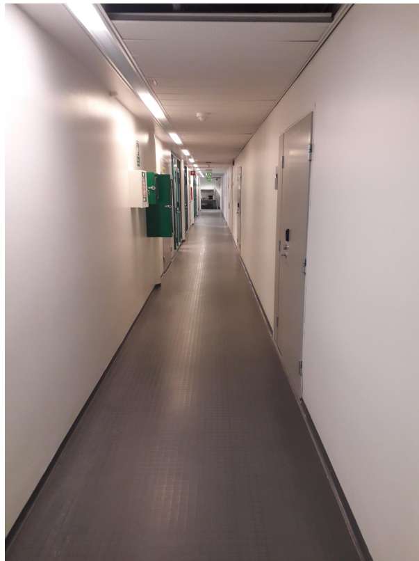
Figure 4. The corridor where LCX cables with adjacent antenna elements were installed behind the white roof (wool) materials. Antennas and cable openings were directed downwards providing energy to corridor and rooms on its two sides.
