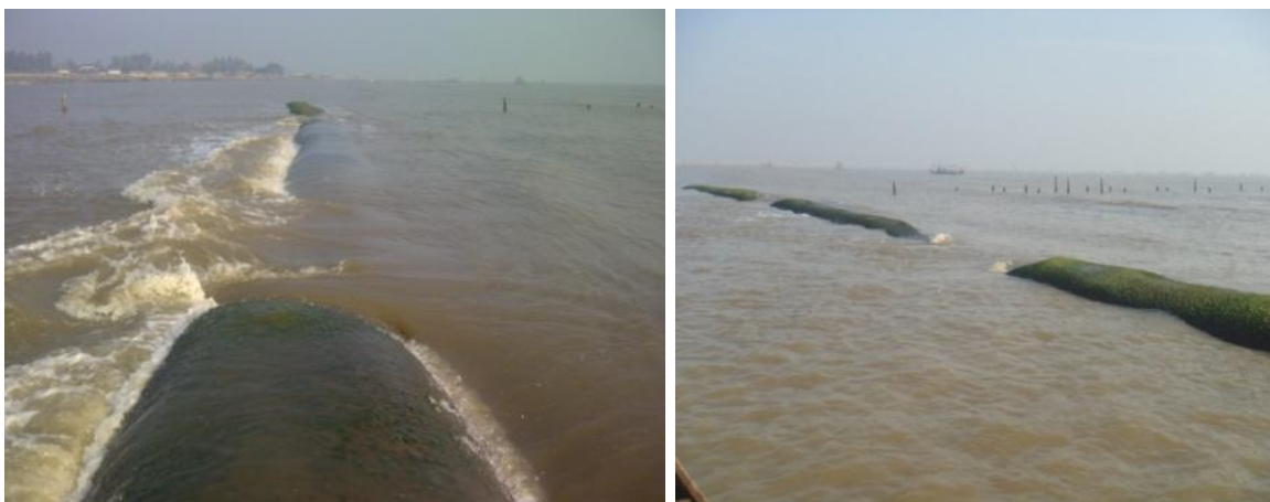
Fig. 3. LCB geotextile tube in Tanjung Kait Beach (Sulaiman et.al., 2012).
