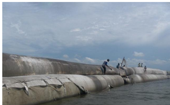
Fig. 8. Two stacking geotextile tubes at Pusong beach, Aceh (Sulaiman et.al., 2012)
