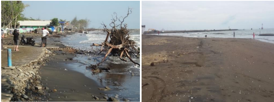
Fig. 6. Sigandu Beach, Before and After LCB Installation (Sulaiman et.al.,2015)
