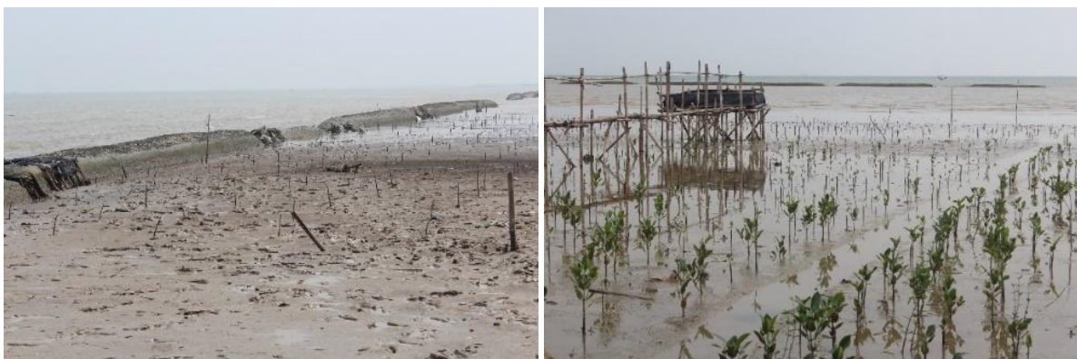
Fig.7. Sedimentation Behind LCB at Pasir Putih Beach, Karawang (MMAF, 2016)
