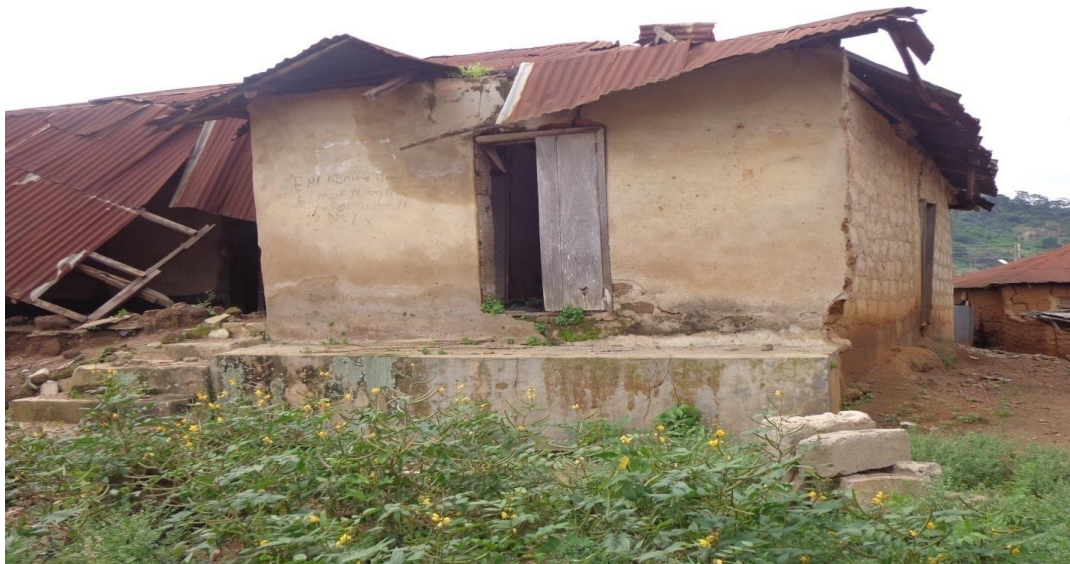
Figure 4: Building that fall with 1km radius damaged by the effects of stone blasting in Akure-Ado axis
