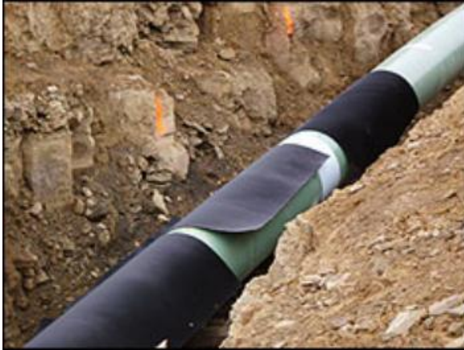
Figure 2: Pipeline insulation for corrosion protection [protectionengineerings.com]
