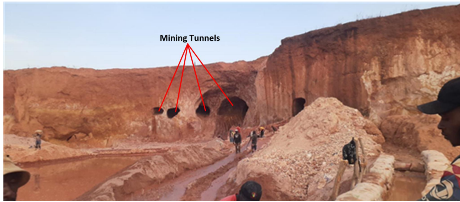
Figure 10. Guratopp Mine Sites Showing the Mining Tunnels
