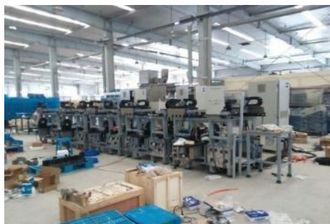
Figure 8. Bent tube polishing production line
